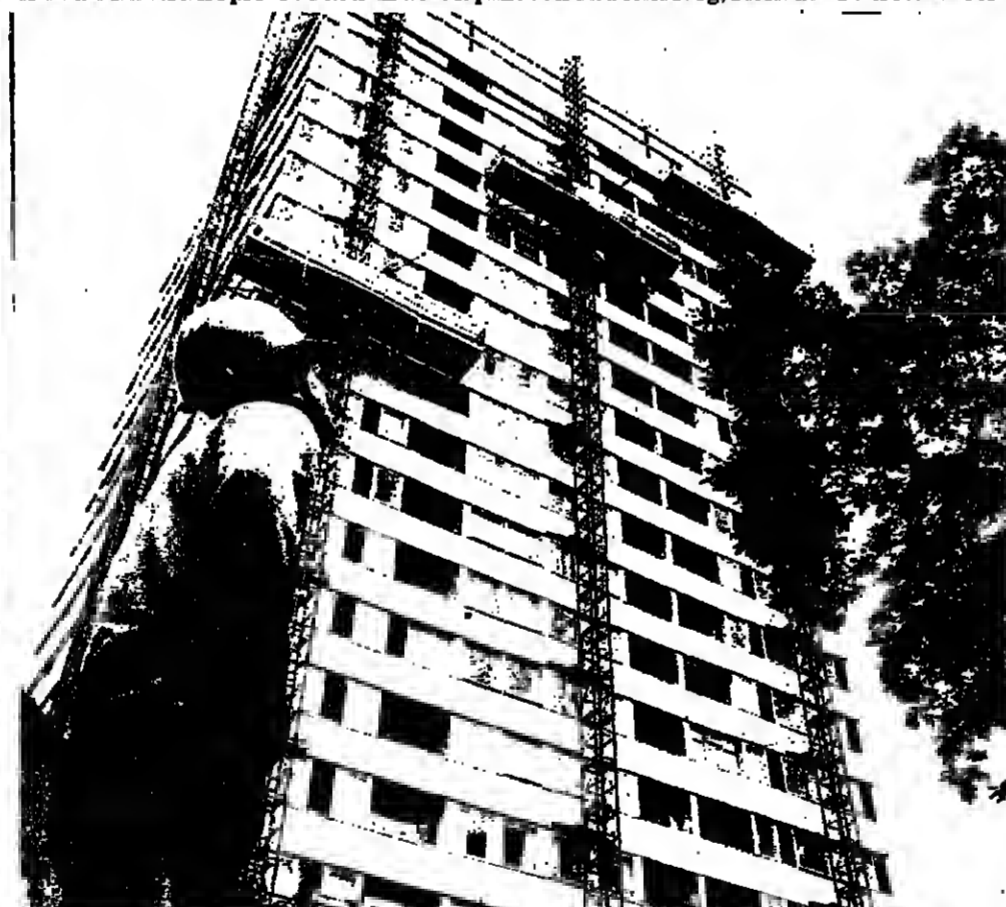
MODERN ELEVATORS: A ramp is not always a practical proposition for a disabled person, so, above left, a scissor lift by Becker provides easy access where an obstacle previously existed. Center, a rack and pinion driven climbing work platform called the Aliclimber runs on steel lattice masts fixed to the building and can be as high as 52 feet. Right, elevated parking enables two cars to park in one space.
